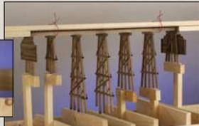
This photo shows how to support the 'sill footers'. Use C-clamps to temporarily position the supports and allow adjustments. Glue and use drywall screws for permanence.
